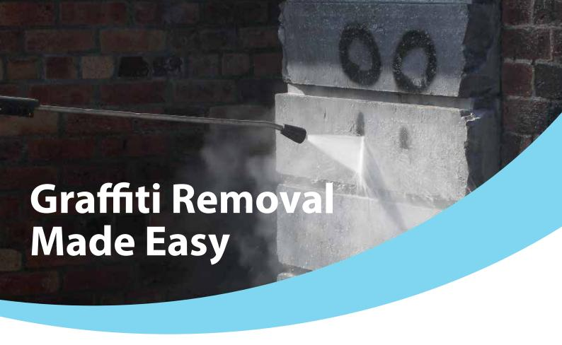
GraffGo® Self Release (SR) is a single pack, anti-graffiti coating that is used to protect infrastructure from graffiti and provide easy removal of graffiti using only water. GraffGo® SR can be easily applied by roller, brush or airless spray to porous and non-porous surfaces.
